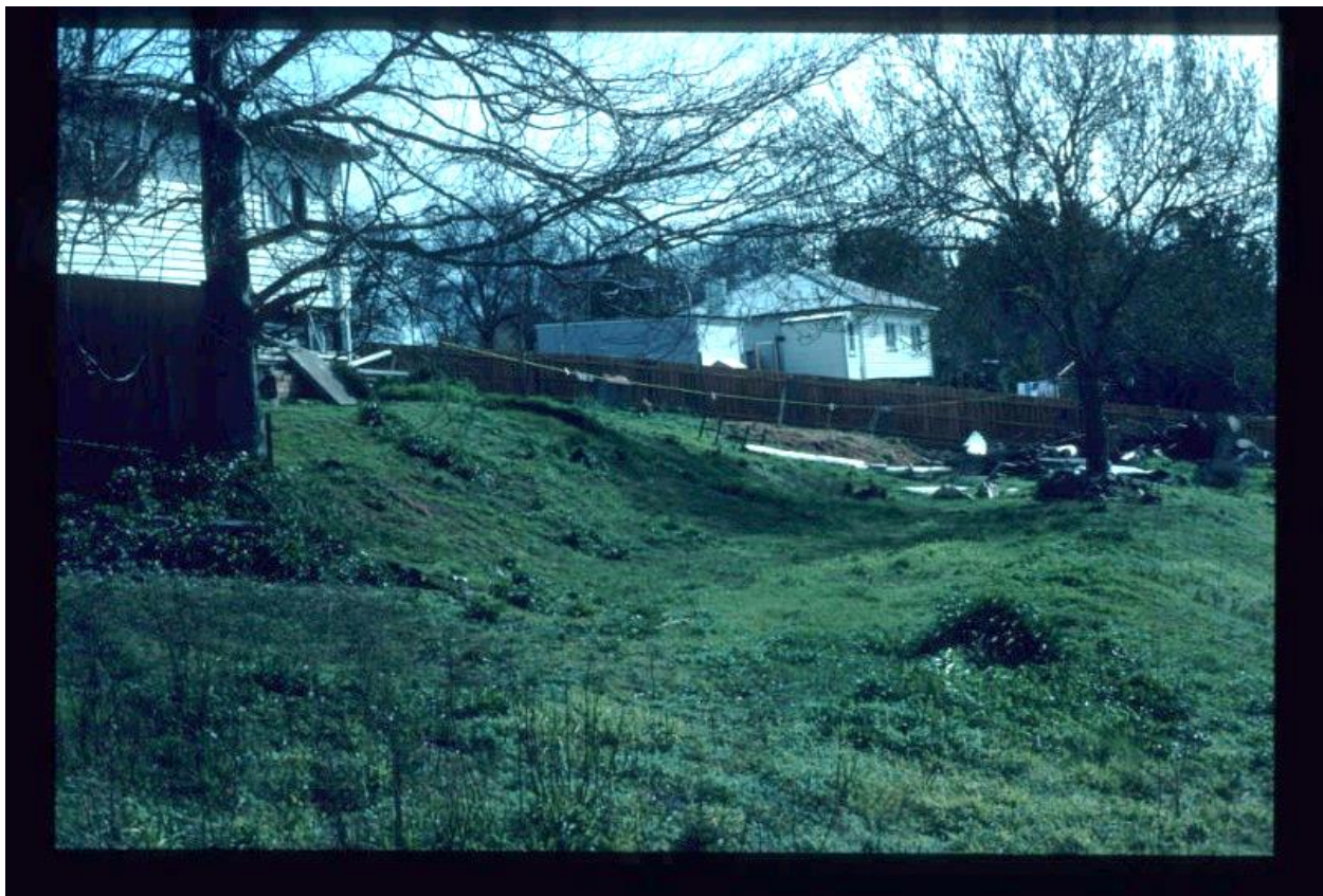
Figure 7. Gisborne Shelter Shed, c.1992 (Heritage Victoria)
