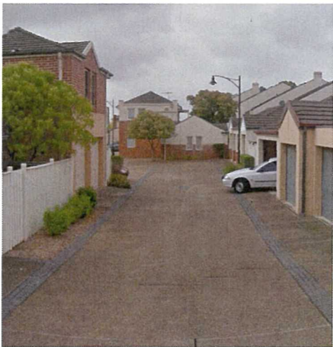
Exposed aggregate concreting with stone detailing Hunterford, NSW
