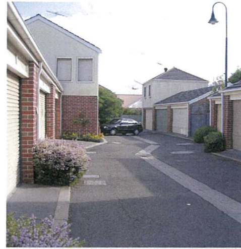
Articulated Lane breaking gun-barrel effect Kenningson Banks, VIC
