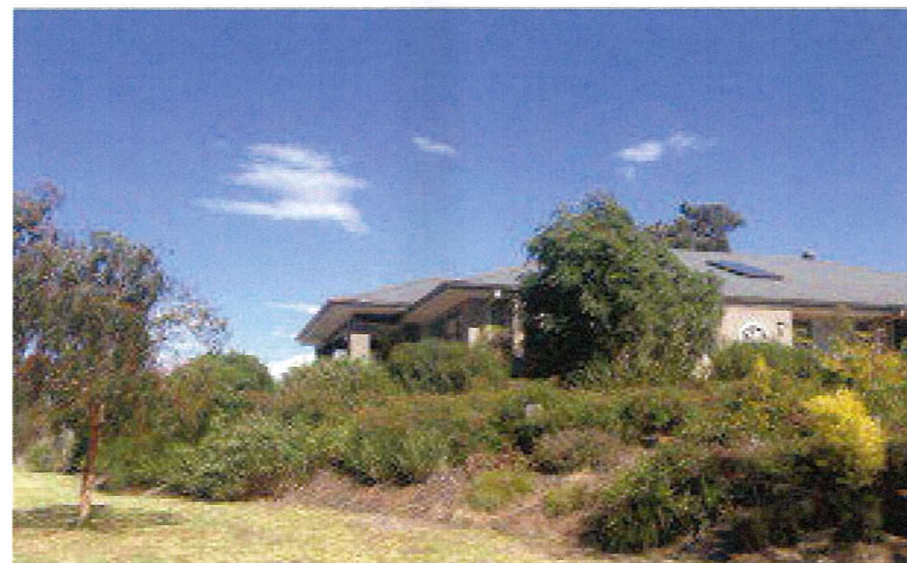
Dense native planting a low maintenance boundary treatment for residents and create clear public and private separation
