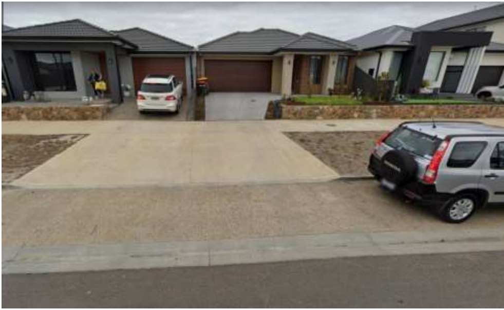
Figure 25 Containment of 1 in 1 million year event flow depth and 600mm freeboard via retaining walls at the front of lots (image at Riverglen Dr within the Greenvale Reservoir catchment)
