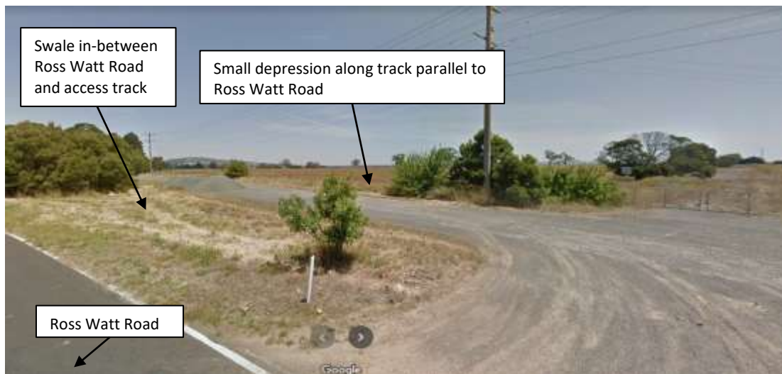
Figure 10 Depression parallel to Ross Watt Road (looking south)
