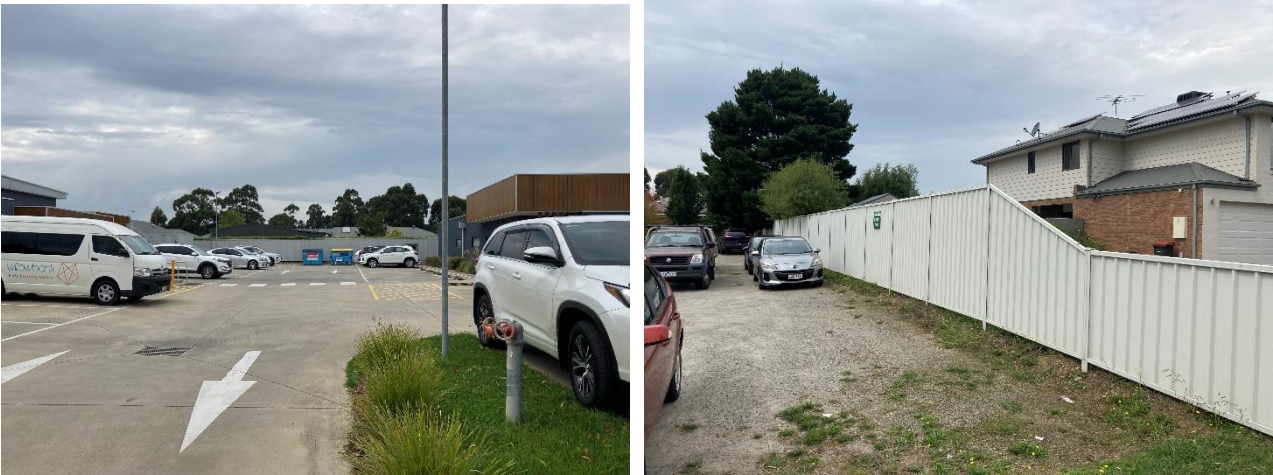
Figure 19: boundary fencing surrounding childcare centre and osteo
