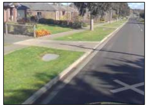
Figure 2 street view - drain intake
