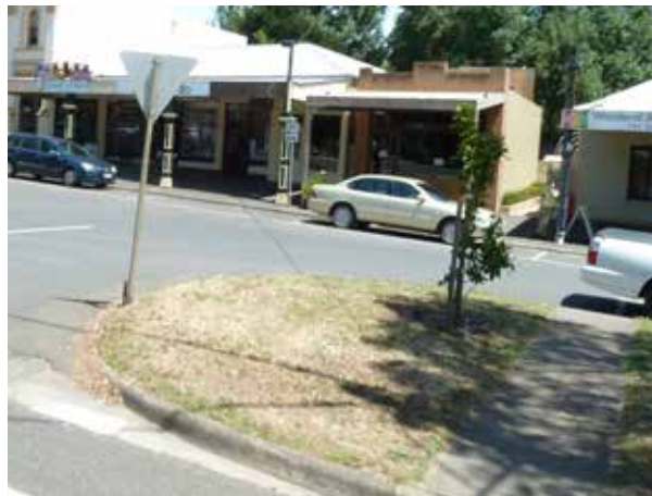
Medians would benefit from upgraded landscaping and formalised pedestrian refuges
