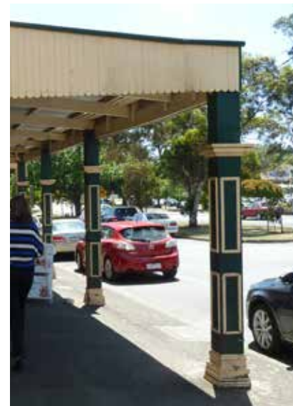
Post-supported verandah, heritage detailing
