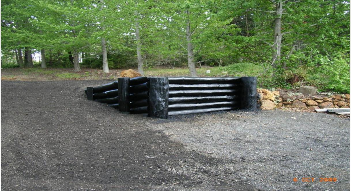
Is used in a number of ways and comes in several designs, from simple as indicated above or have higher sides for difficult to load horses. When set at the right height the truck or float backs up to the loading ramp, lowers the tailgate and horses can then be led in to the vehicle.
