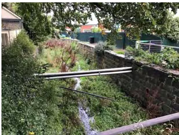
Bluestone rockwork and drains within Bunjil Creek.
