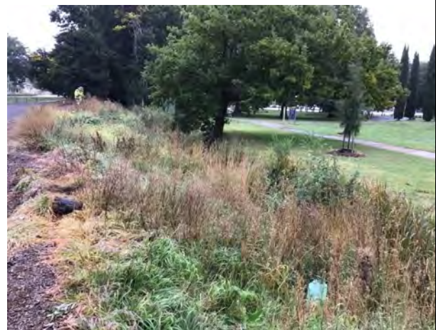
Partial revegetation works within Bunjil Creek
