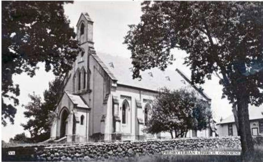
GMMDHS Photo D2260 12A5, Presbyterian Church 1950s with rock wall
