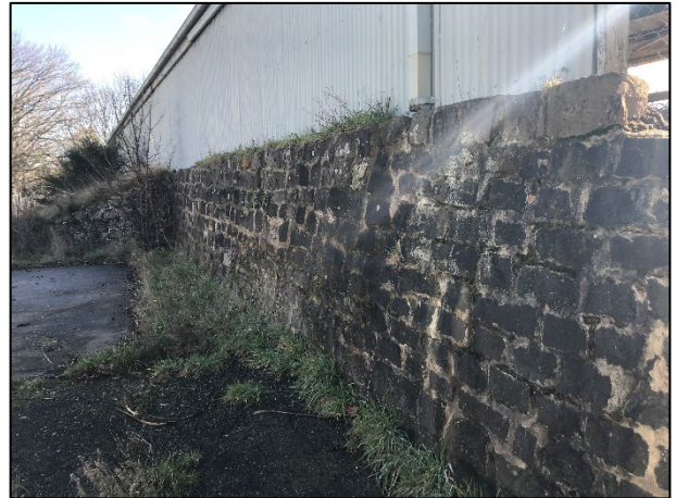
Figure 6. Southern side of grandstand with bluestone retaining wall (GJM Heritage/Frontier Heritage, July 2018)
