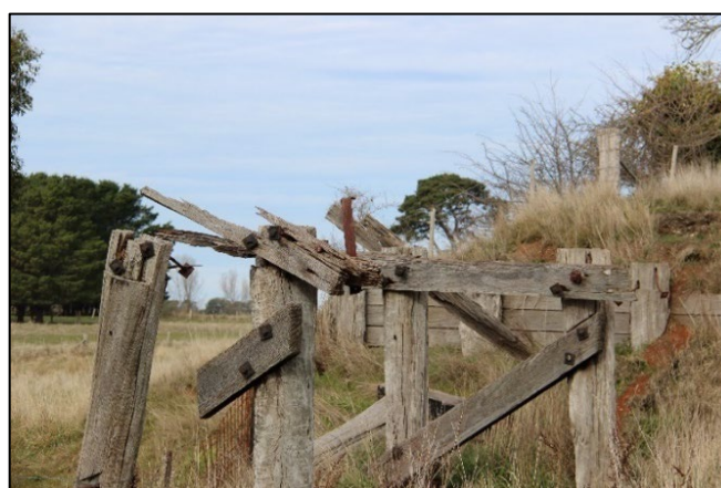
Figure 18. Remnant timber trestle bridge (GJM Heritage/Frontier Heritage, July 2018)
