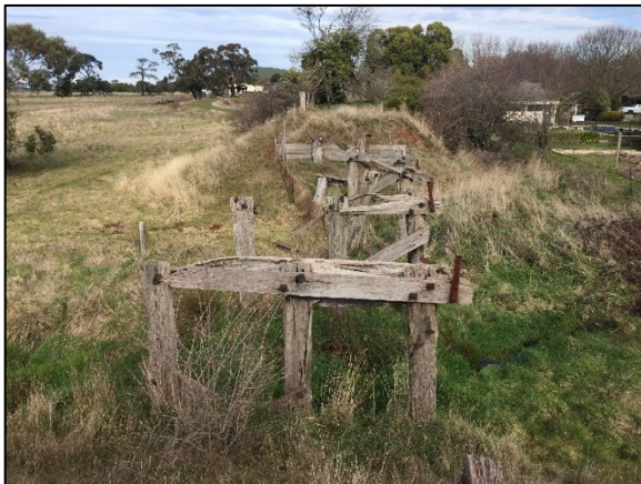
Figure 21. Remnant of timber trestle bridge (GJM Heritage/Frontier Heritage, July 2018)
