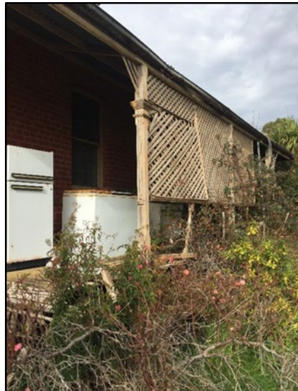
Figure 10. Verandah posts and lattice work (GJM Heritage/ Frontier Heritage, July 2018)
